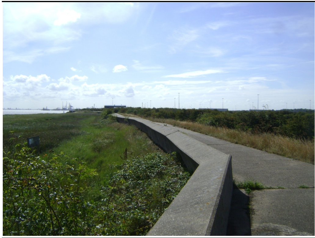
Figure 6.10 Estuary Flood Defences at Site
